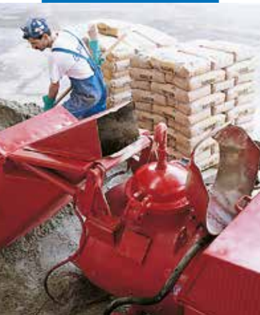
Mixing Topcem with an automatic pumping unit
