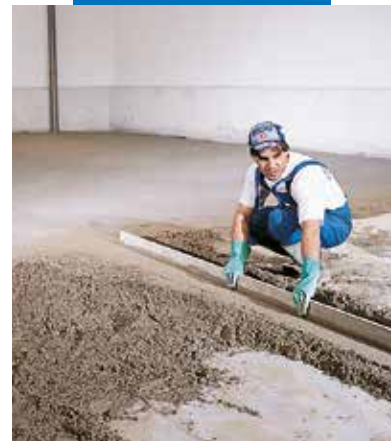
Preparing a levelling strip
